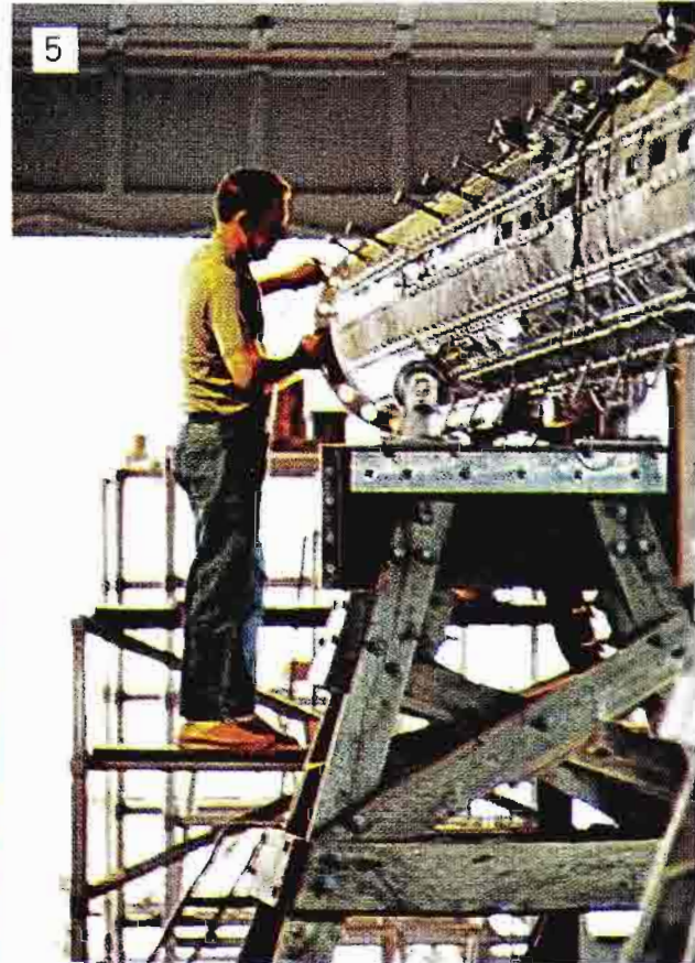
(5) Assembling one of the largest Pylon Antennas ever built. It will provide a base for a large Super Turnstile antenna in a stacked antenna arrangement.
